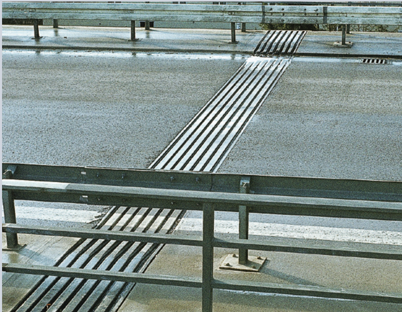
Girder Grid Joint type D 560
