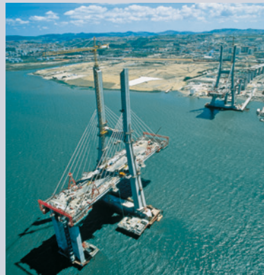
Vasco da Gama Bridge, Portugal
