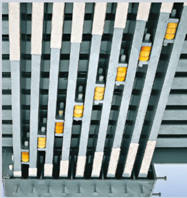
Control of MAURER Girder Grid Joints
