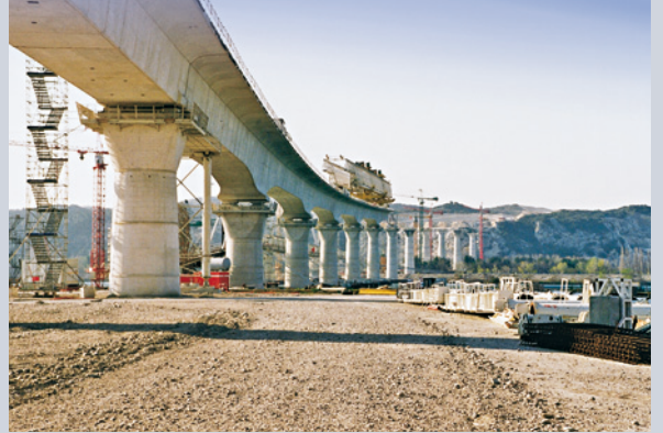
TGV Viaduct, Avignon
