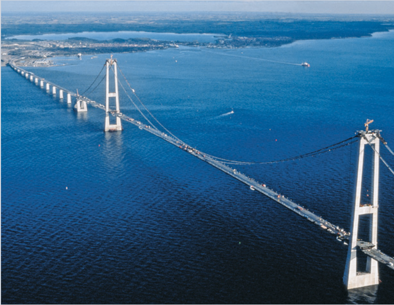
Storebælt East Bridge, Denmark
