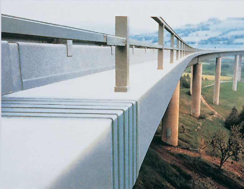
Watertight design of parapet
